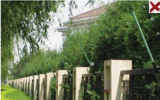
The camera's angle of depression is not wide enough; there are so many trees in the scene. The above mentioned environment is too complex to detect the intrusion.
