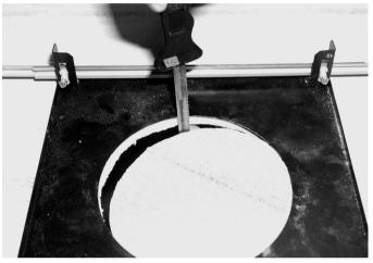
Figure 3.2 Cut Hole in Ceiling Tile
